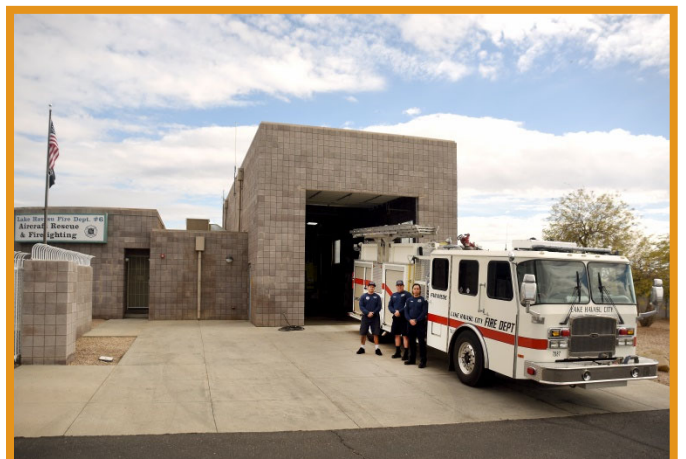
Station 6 | 5600 Hwy. 95 N. 218 calls
