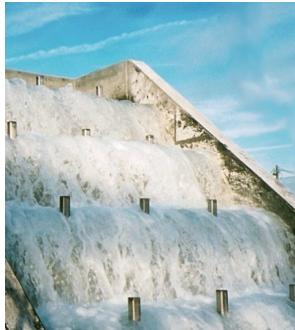
Drinking water flowing into the Lake Havasu City Water Treatment Plant from wells next to Lake Havasu.
