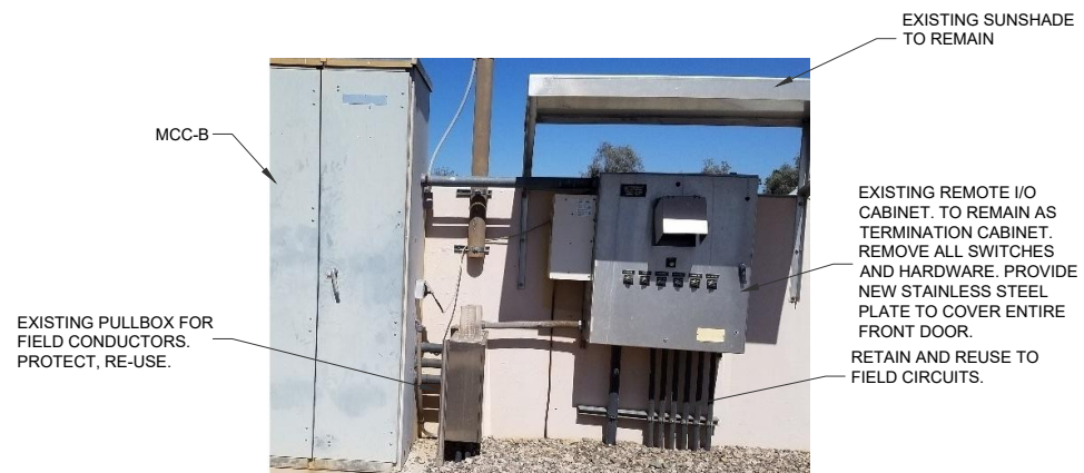
1 PHOTO 1 - EXISTING MCC-B ELEVATION E-402 NO SCALE
