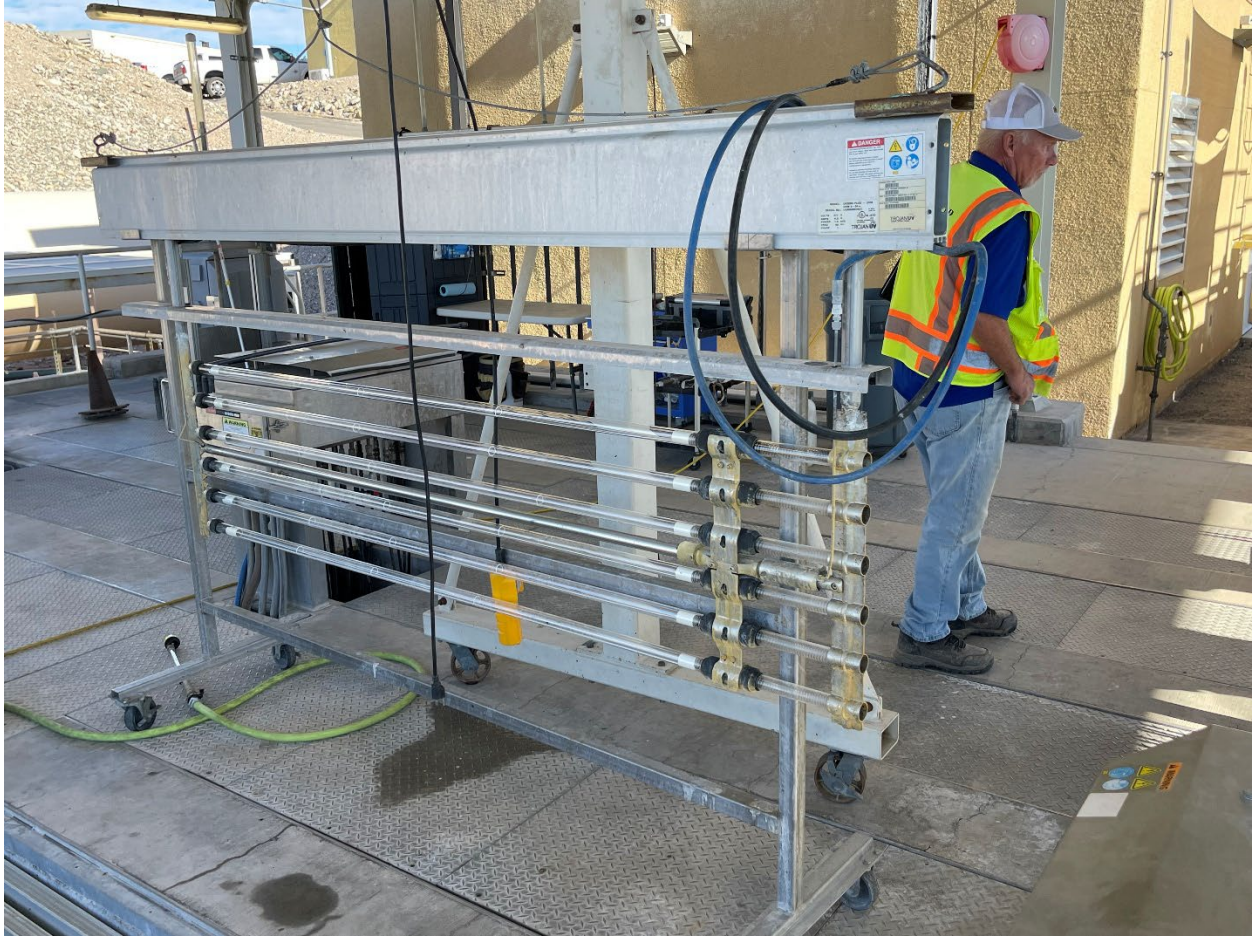
Picture B-7 : Bulb assembly (6 UV bulbs on stainless steel rack with wiring). Installed as groups of six racks. A total of six groups is installed (36 total assemblies).
