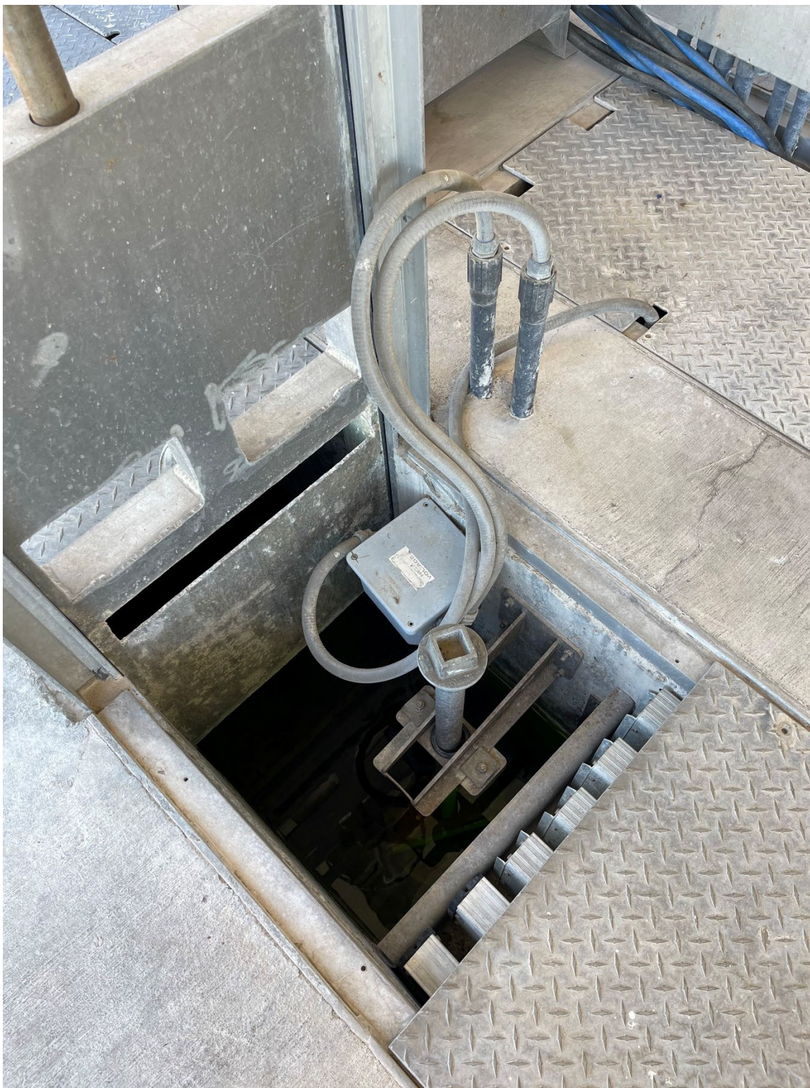
Picture B-4 : Transfer box and cables
