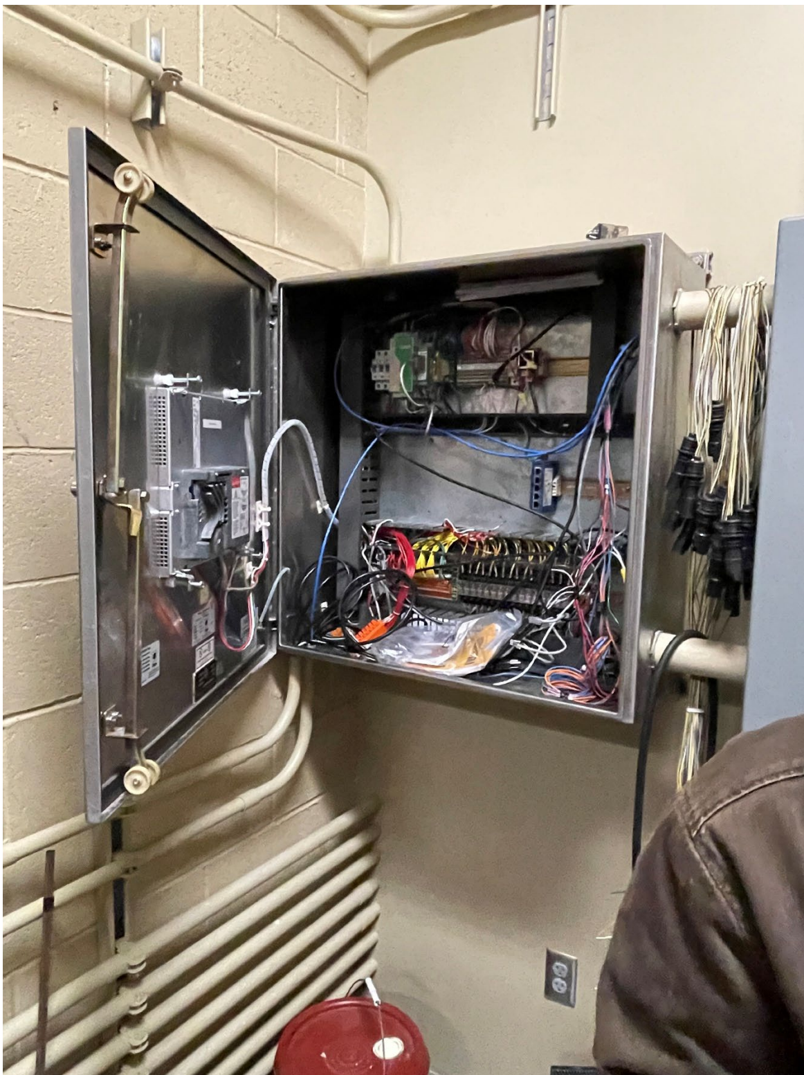
Picture B-5 : Previous controller box (functioning as a junction box)
