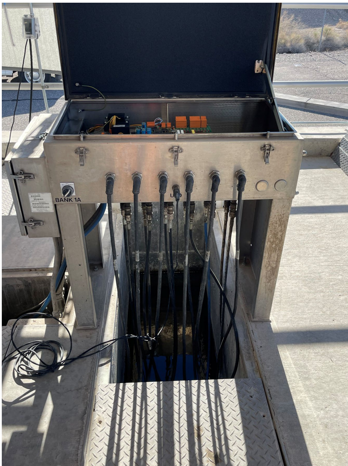
Picture B-2 : Cables from Power Control Board to bulb assemblies.
