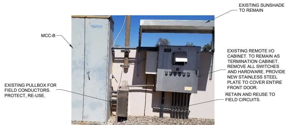
1 PHOTO 1 - EXISTING MCC-B ELEVATION E-501 NO SCALE
