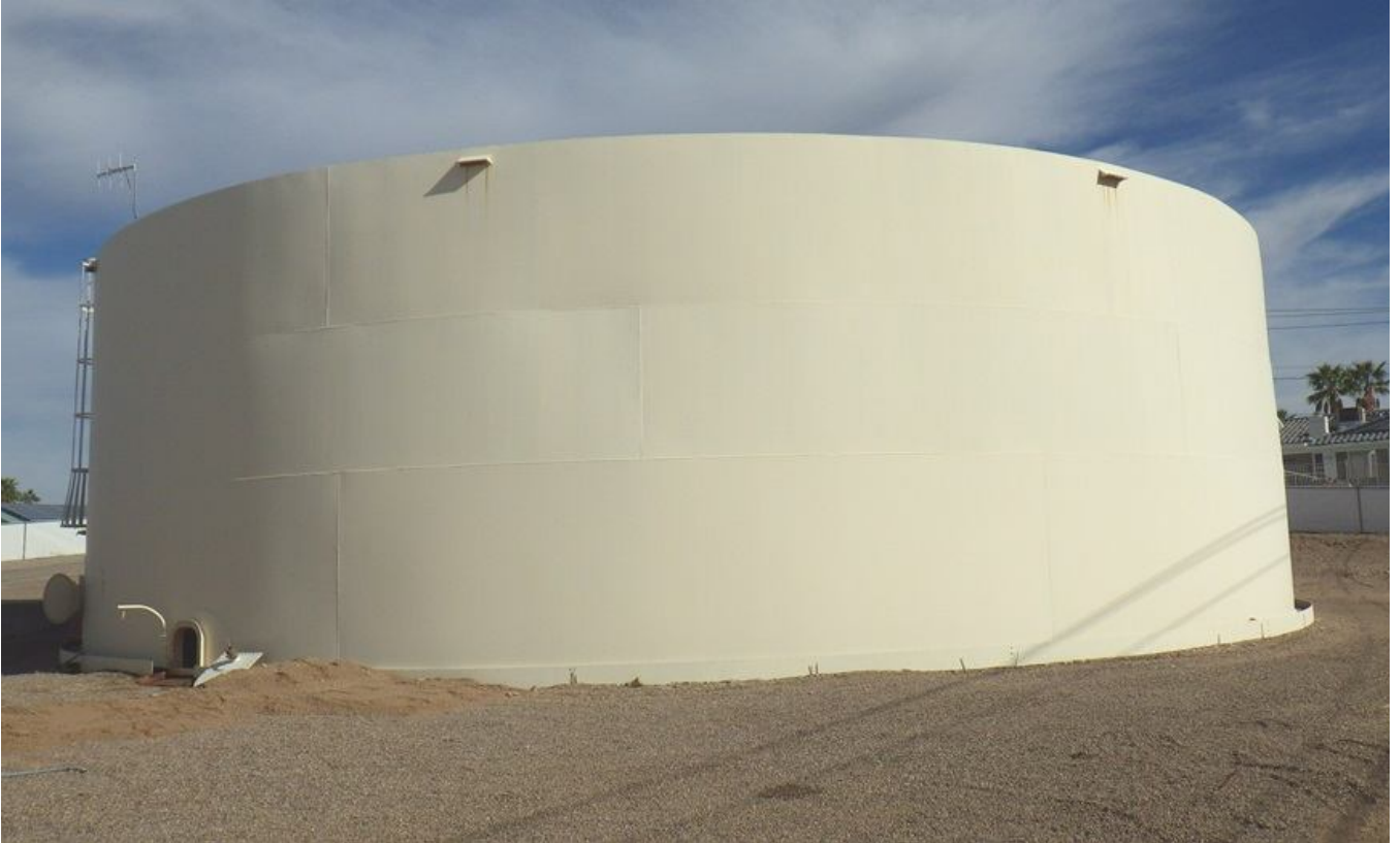
2. Tank and site.
