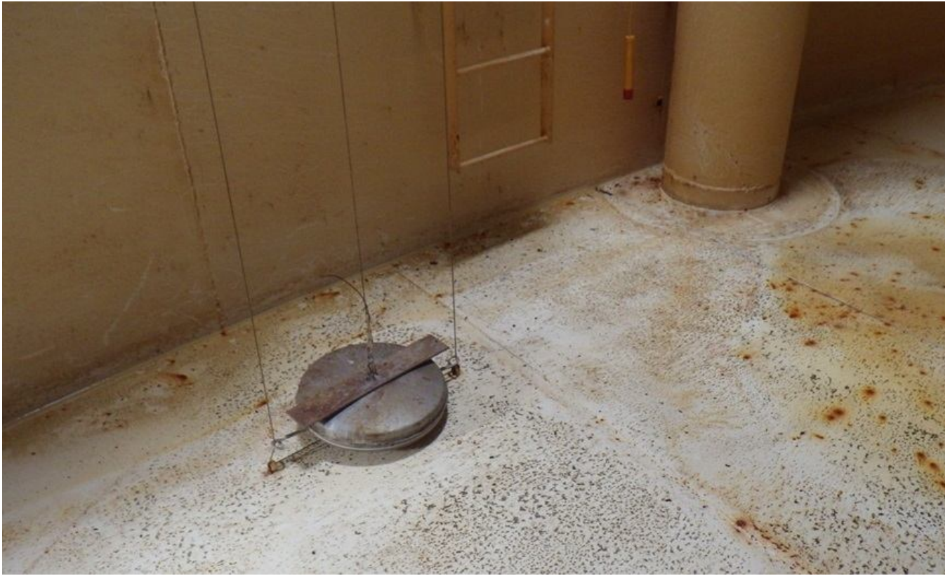
89. Target gage float and cables.
