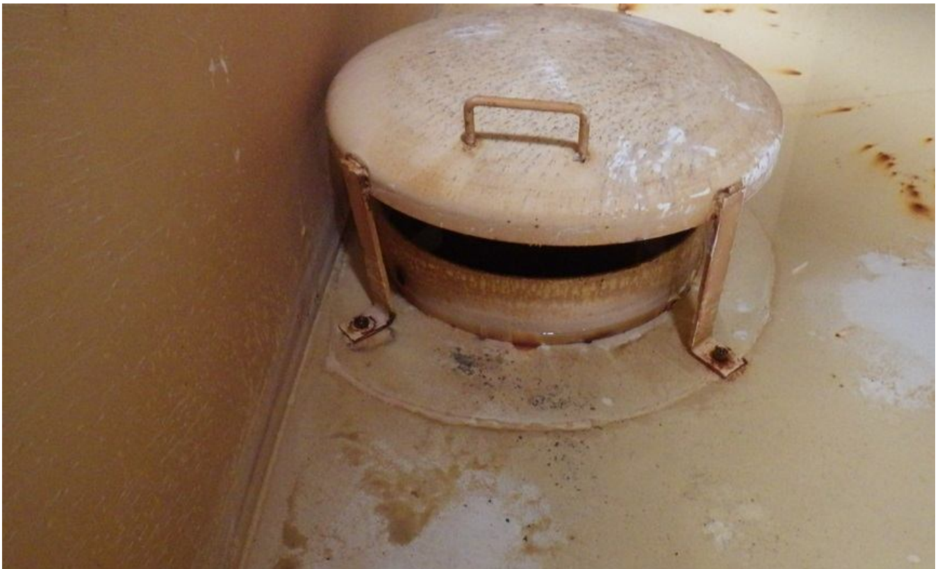
86. Outlet pipe, removable cover, and mud guard.
