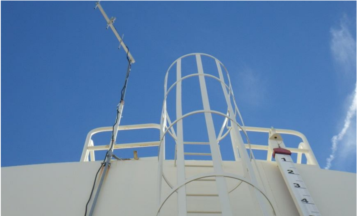
35. Antenna, roof safety railing, ladder safety cage, and target gage.
