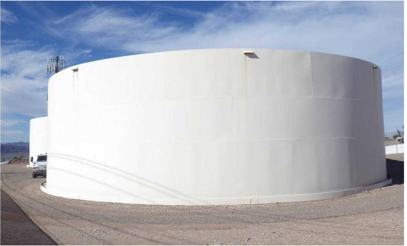
1. Tank and site.
