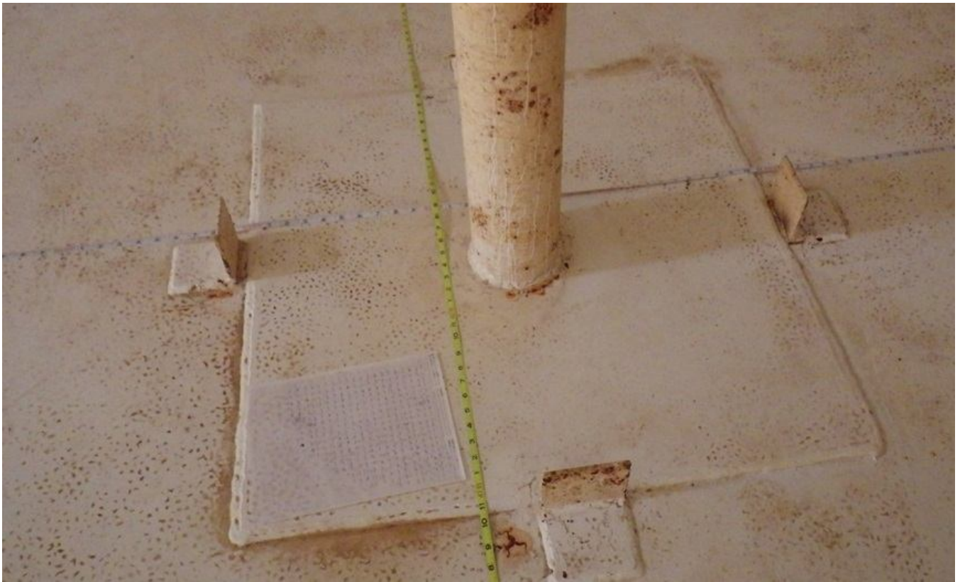
97. Center column base and angles.
