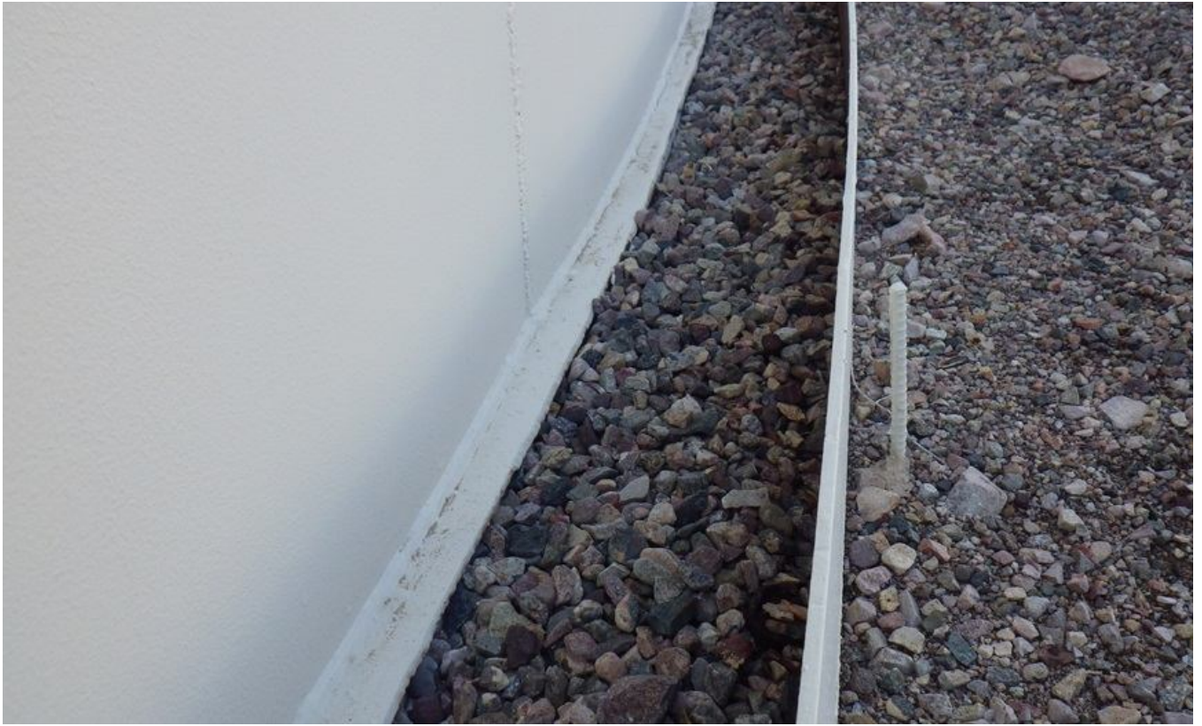
11. Retaining ring around tank. Note rod.
