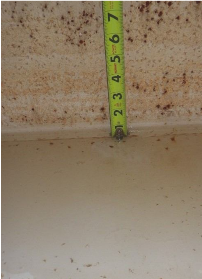
91. Shell-to-floor connection.
