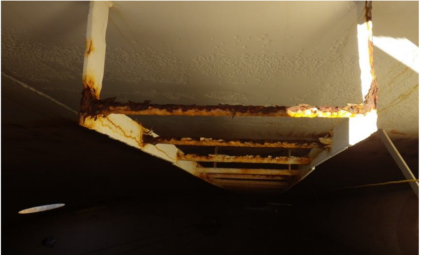
75. Corrosion and metal loss on upper interior ladder.
