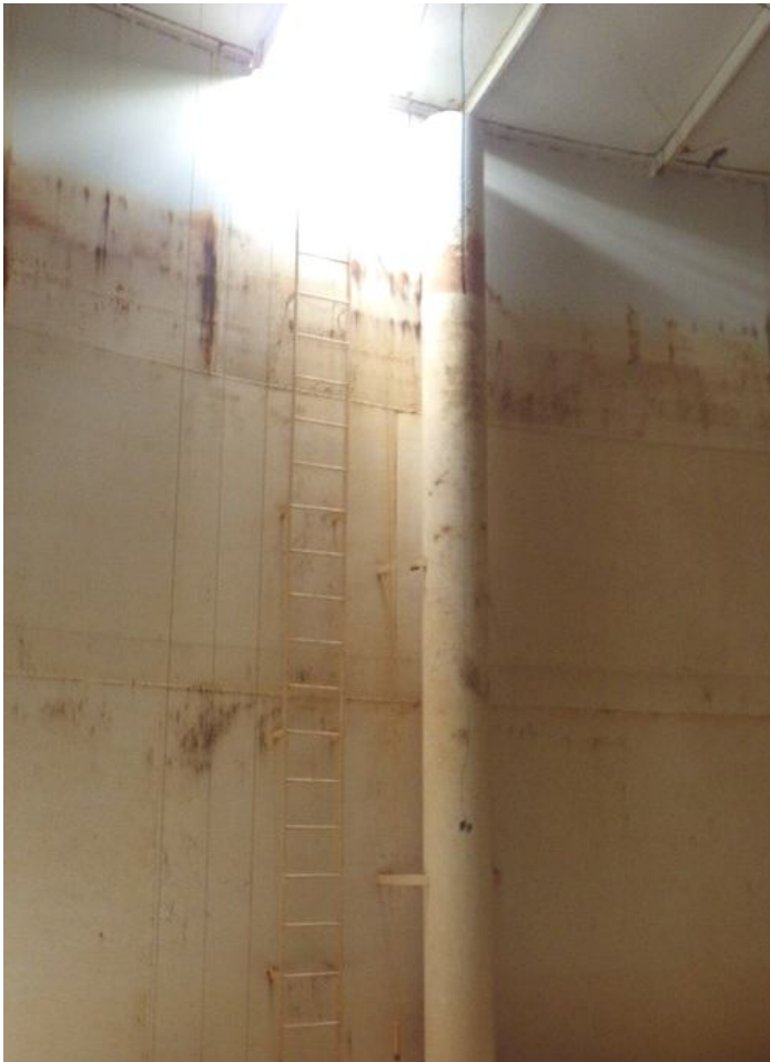
75. Corrosion and metal loss on upper interior ladder.
