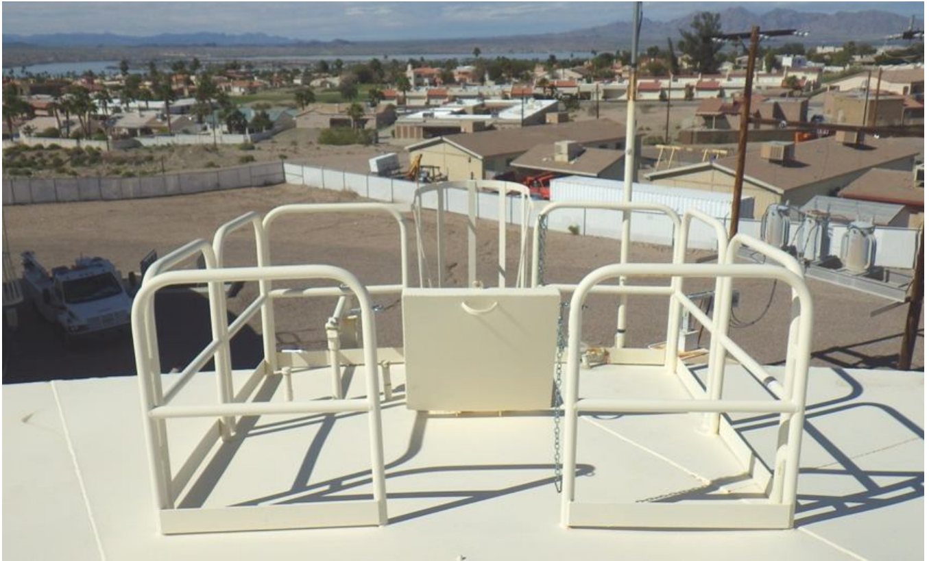
41. Roof safety railing and roof manhole.
