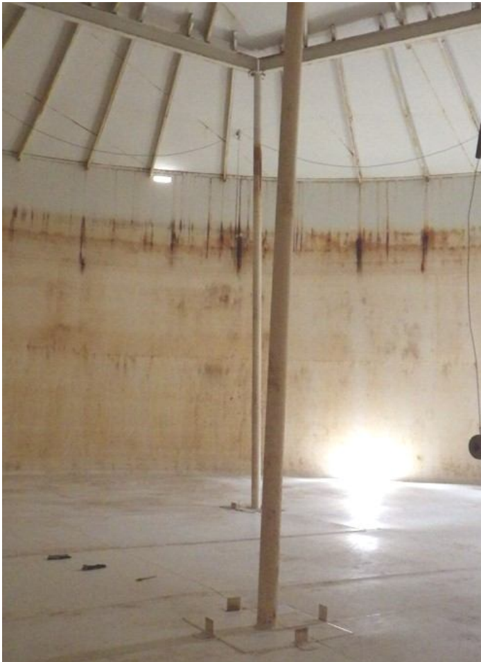
57. Center column, center hub, and inner rafters. Note peeled coating, corrosion, and rust staining.
