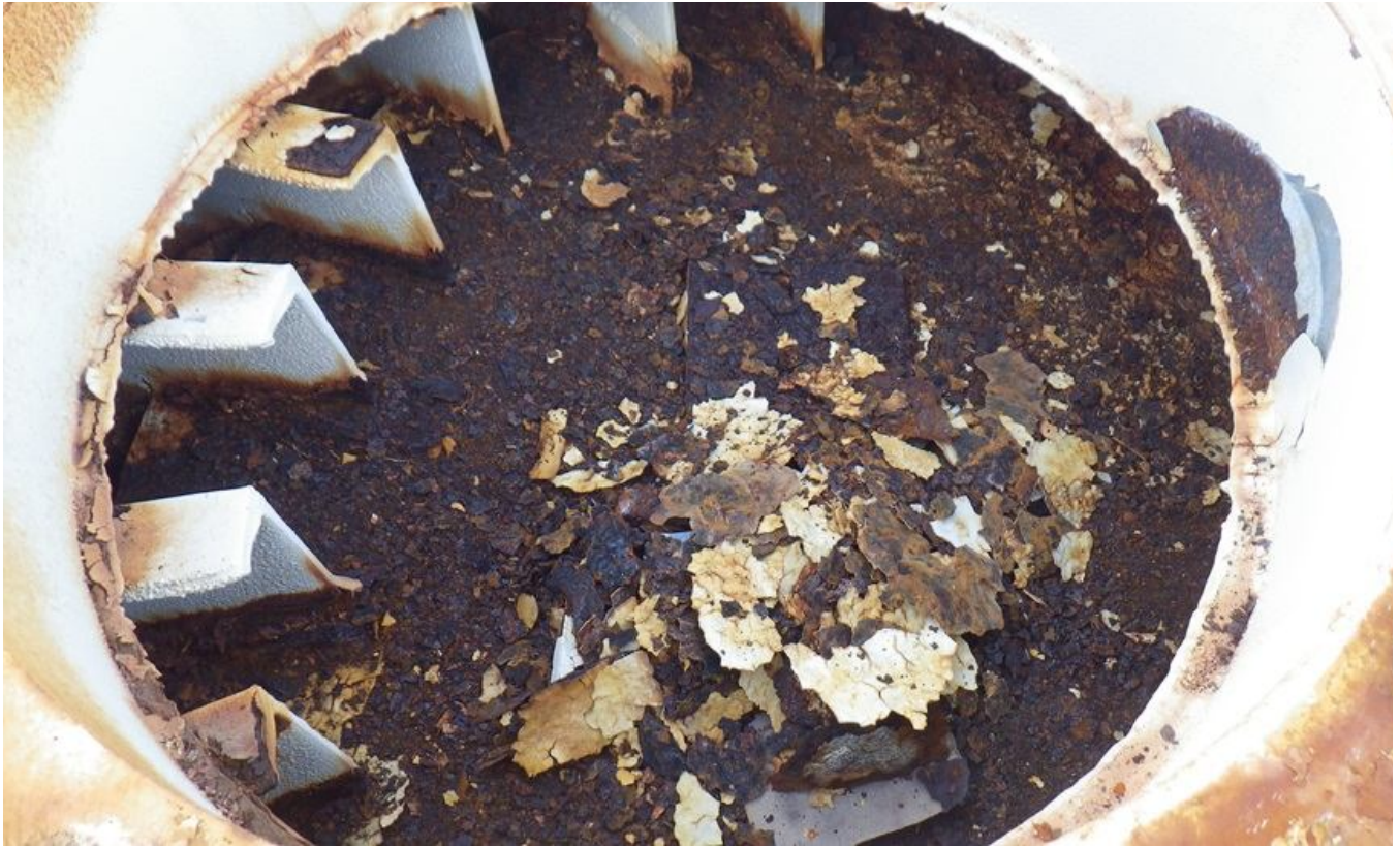
51. Corrosion and metal loss on top side of center hub at removable cover vent.
