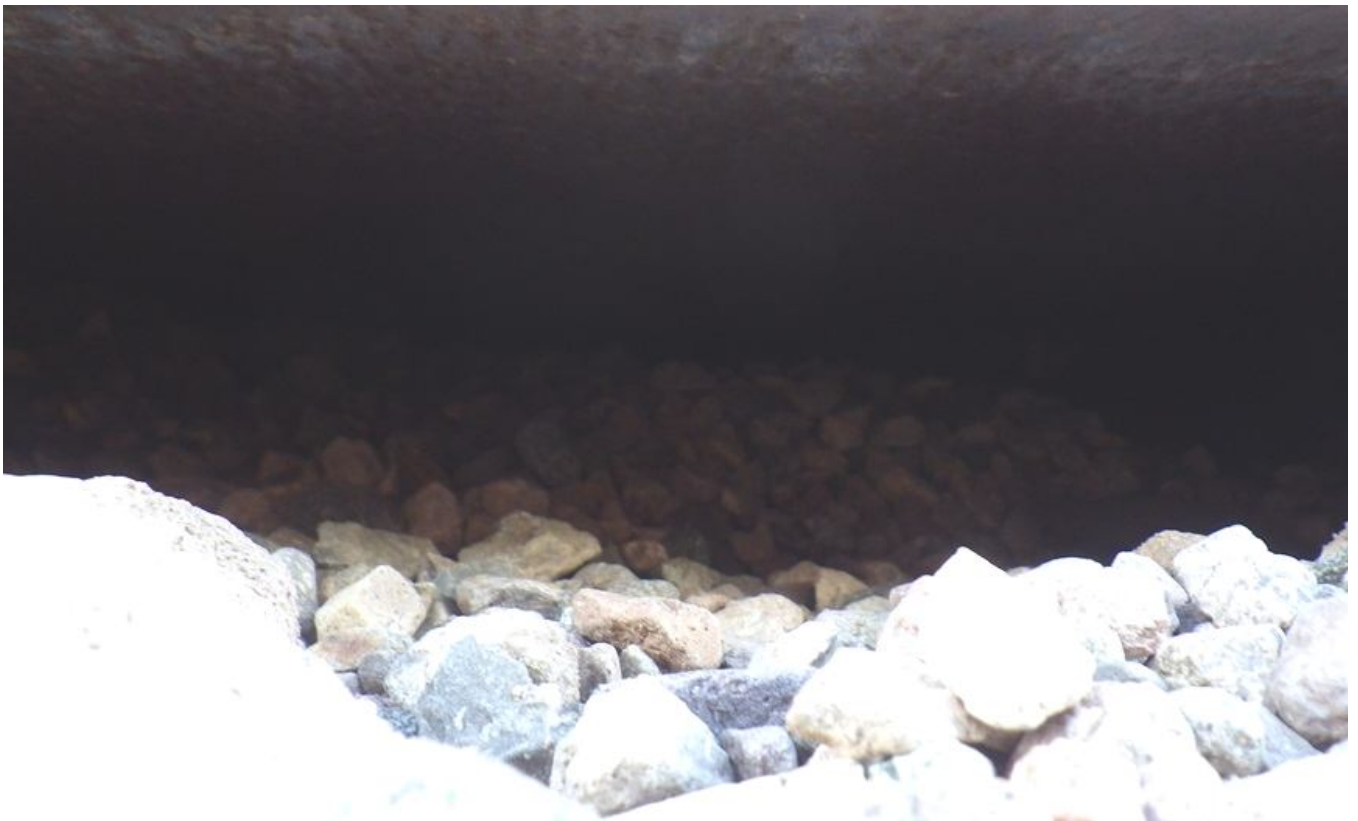
18. Gap between bottom plate and gravel.
