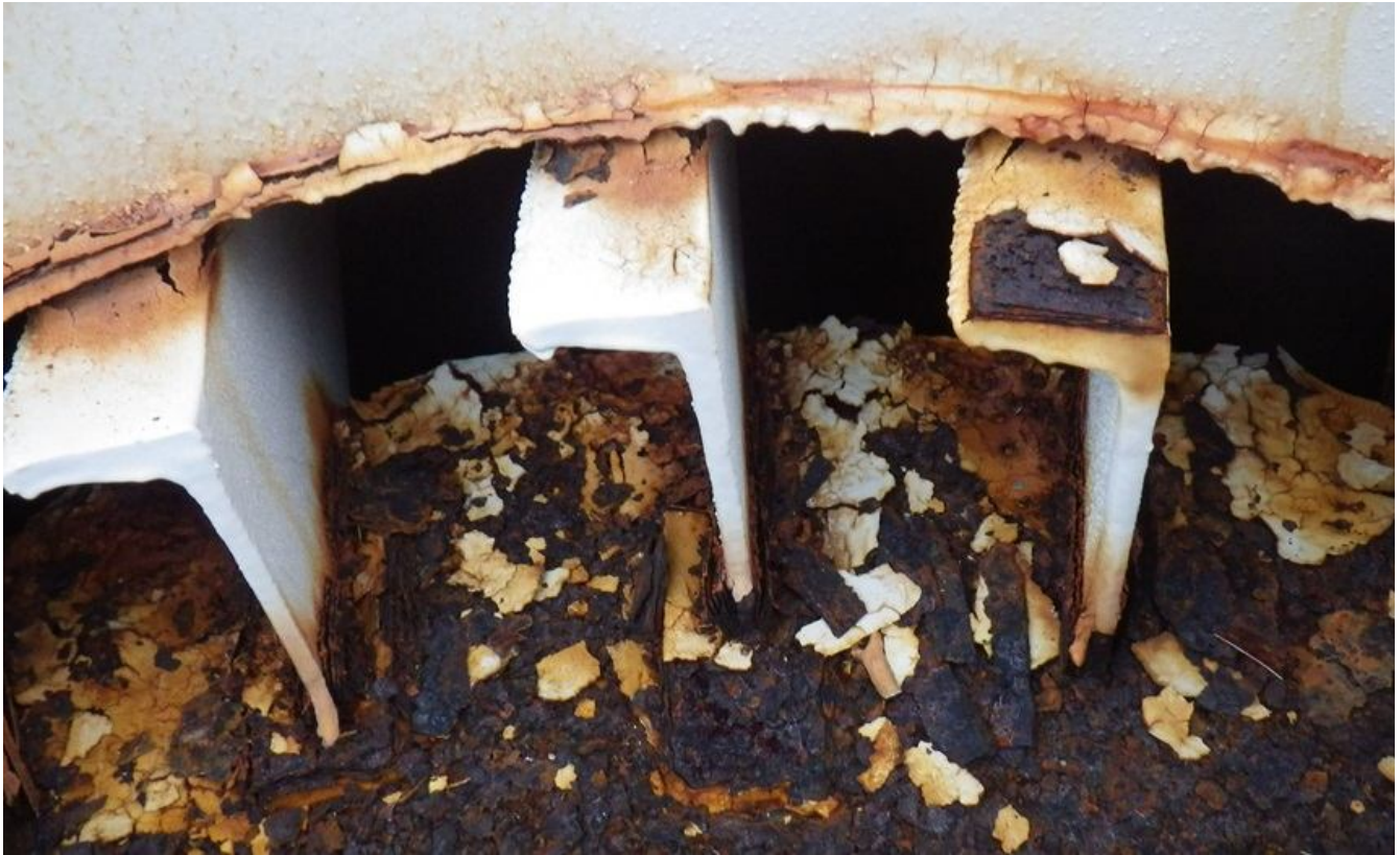
55. Corrosion and metal loss on rafter end and top side of center hub at removable cover vent.
