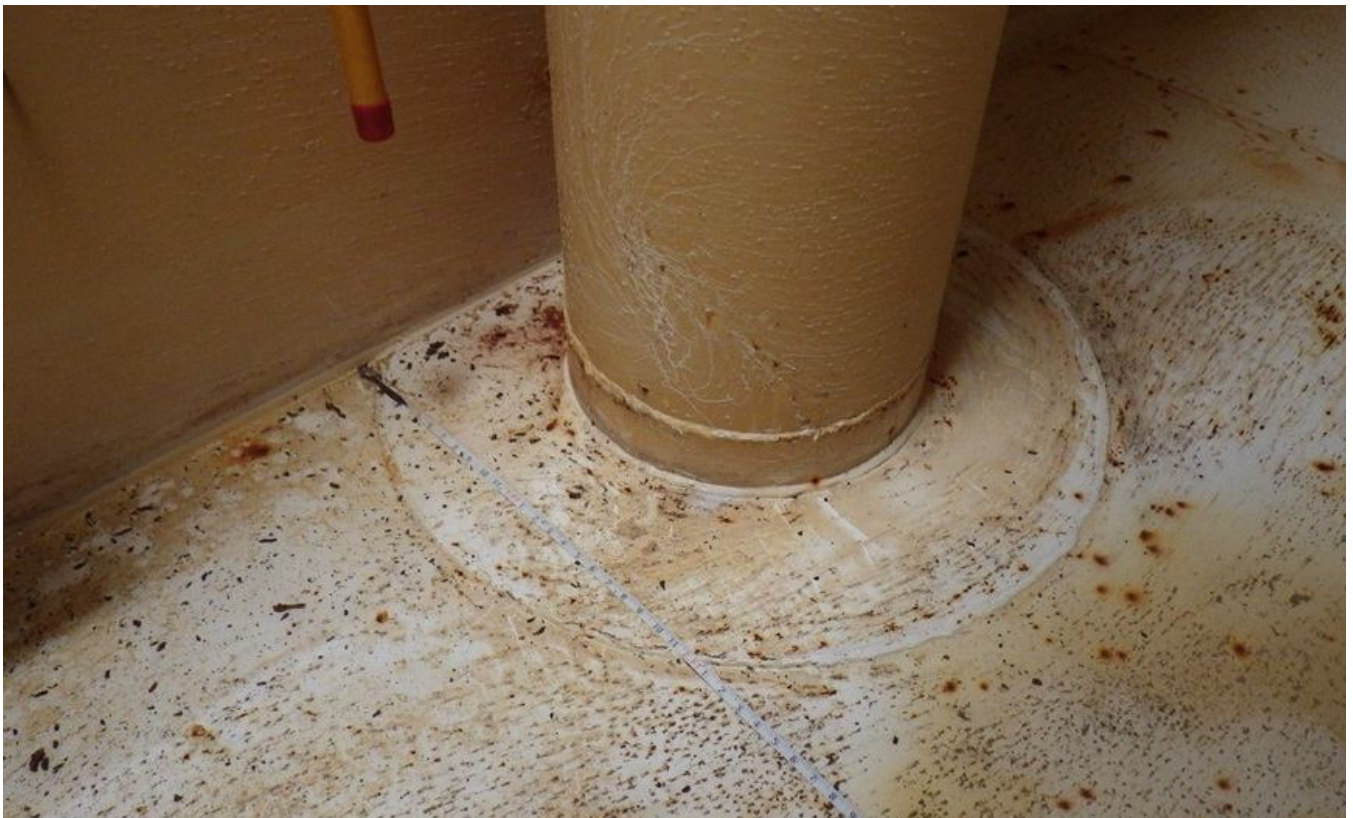
88. Reinforcing plate on floor around overflow pipe penetration.
