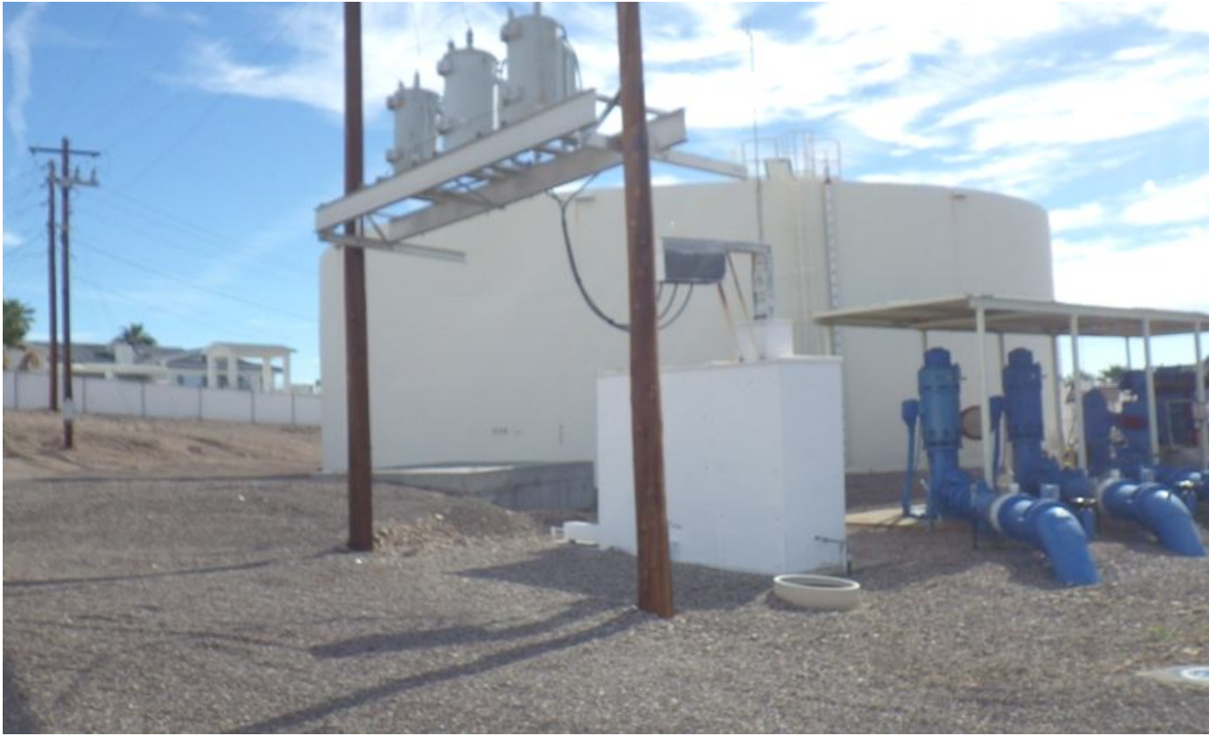
3. Tank and site.
