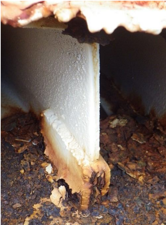
51. Corrosion and metal loss on top side of center hub at removable cover vent.
