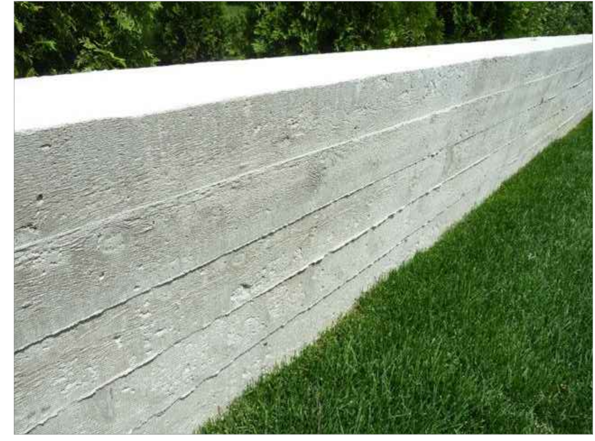
NOTE: BOARD FORM FINISH INTENT AS SHOWN
