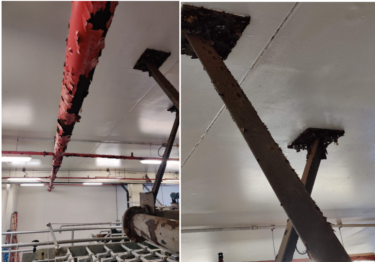
Figure E-7. Hydrogen Sulfide Corrosion on the Fire Sprinkler Piping and BFP Overhead Supports
