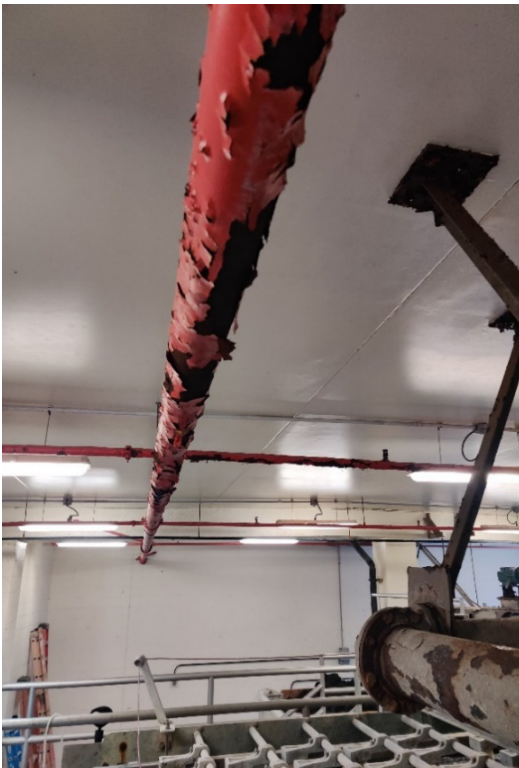
Figure 6-15. Hydrogen Sulfide Corrosion is Observed on the Fire Sprinkler Piping and BFP Overhead Supports
