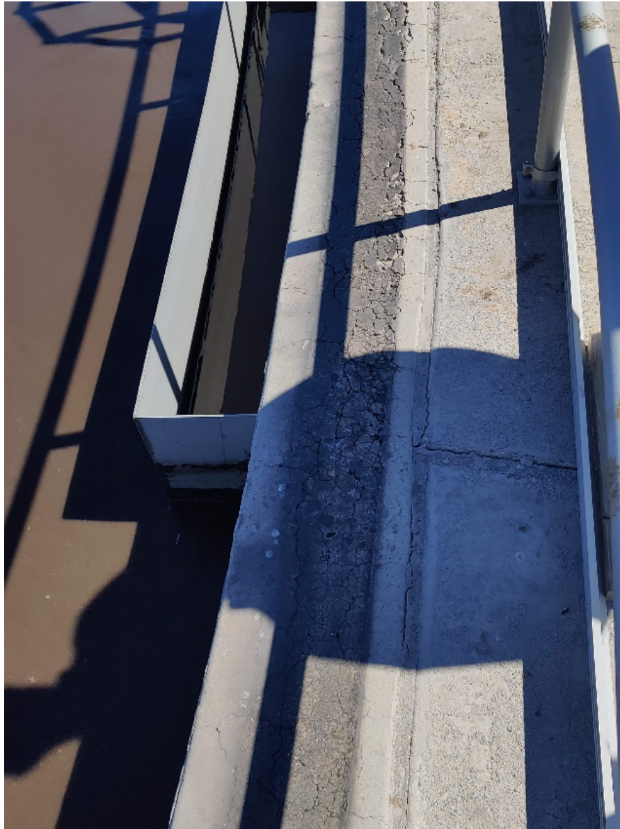
Figure D-7. Cracks Observed on the Edge of the Aeration Basin Concrete Wall
