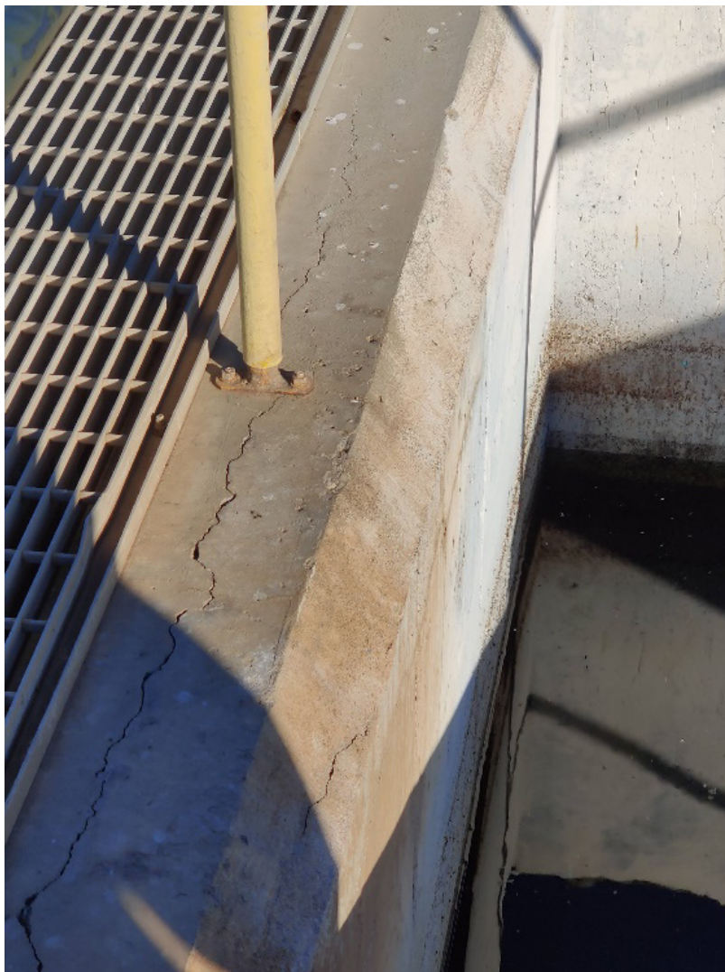
Figure C-7. Cracks Observed in the Concrete Walls of the Sand Filter
