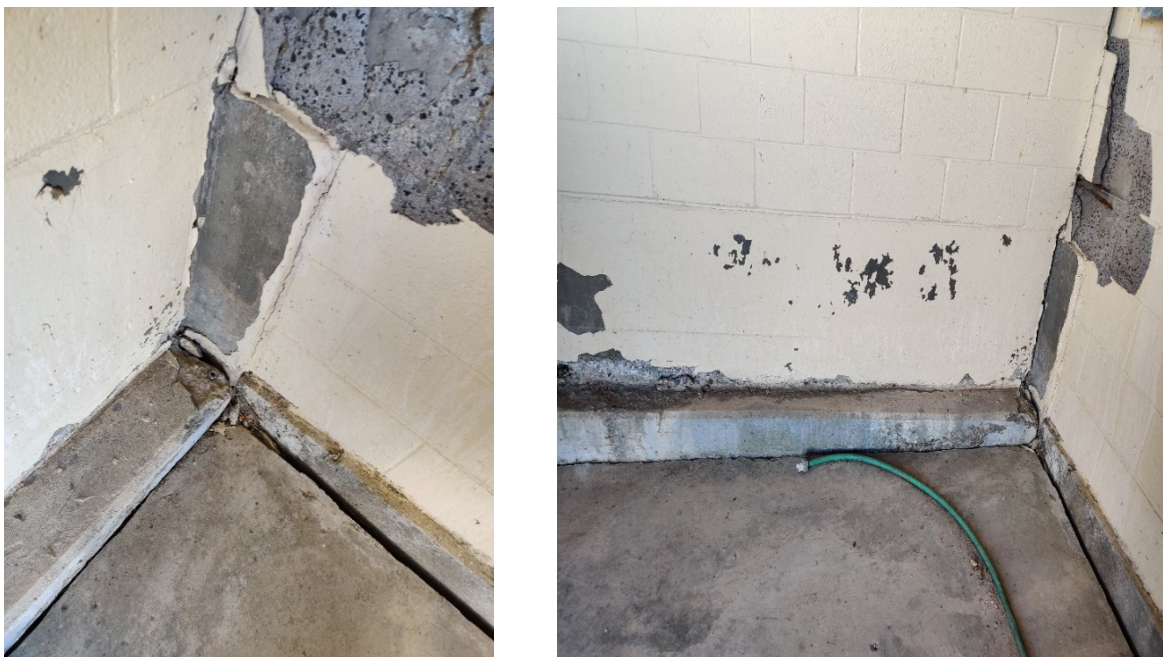
Figure 6-6. Cracks Observed in the South Wall of the Headworks Building
