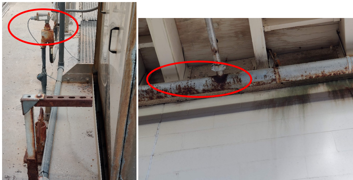
Figure E-3. Typical H 2 S Corrosion of the Electrical System and Fire Sprinklers
