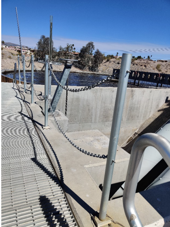
Figure 6-11. Chain Railing Installed at the Top of the RAS Sump Pit; RAS Pumps are Located to the East
