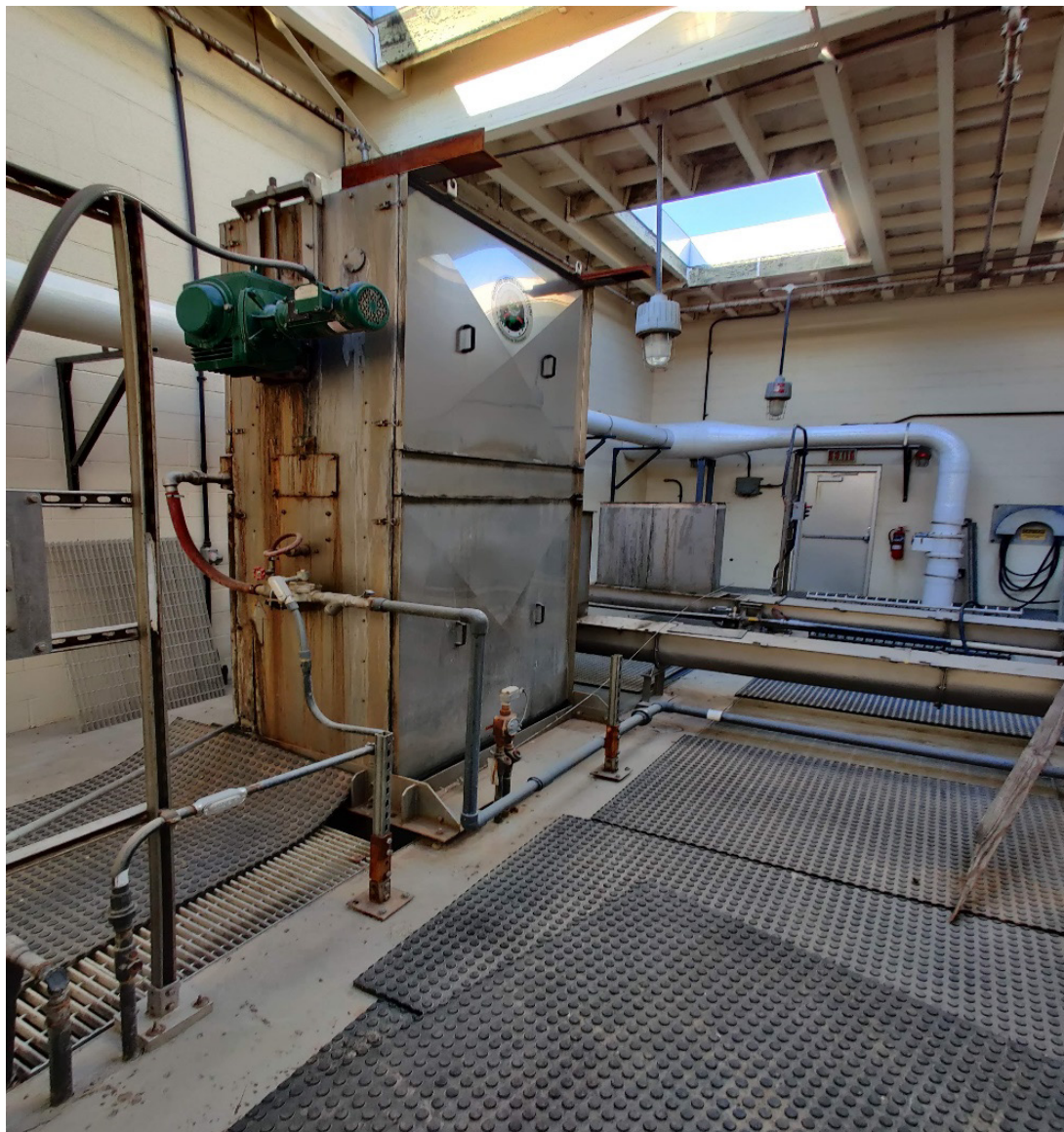
Figure 6-13. Screen Enclosure Showing Signs of Corrosion
