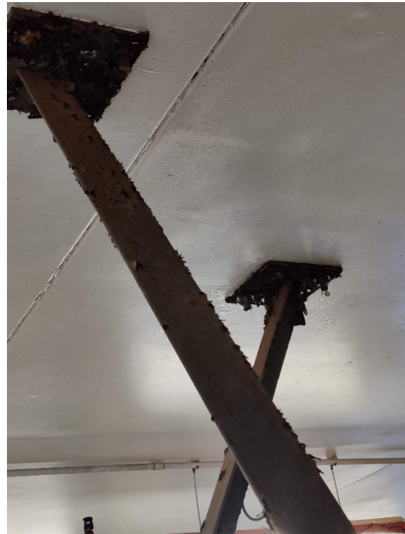
Figure 6-15. Hydrogen Sulfide Corrosion is Observed on the Fire Sprinkler Piping and BFP Overhead Supports
