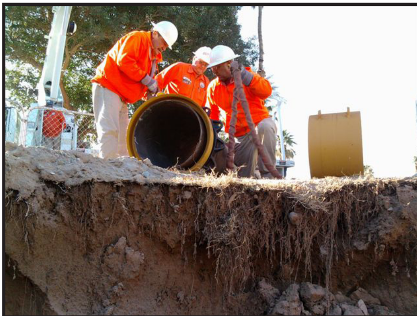
Repairing a reuse line at London Bridge Beach Park
