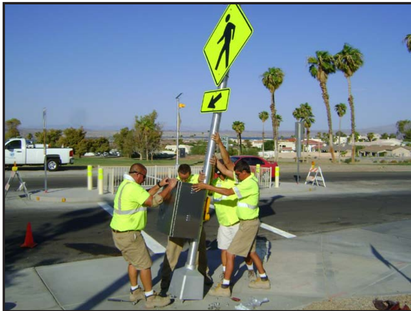
Streets Crew Installing Solar Walk Sign
