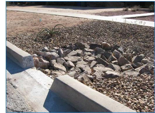
A rock apron protects against soil erosion where curb cuts draw stormwater into bioretention areas.
