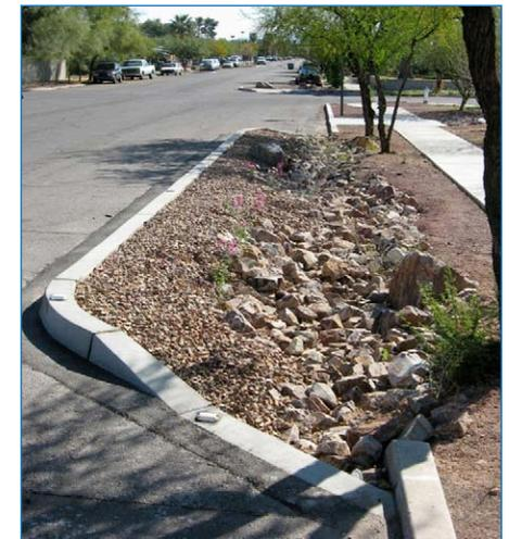
In this just-installed chicane, 4"-8" rock is used in the channel where stormwater will flow rapidly, and 1" gravel covers upslope areas.
