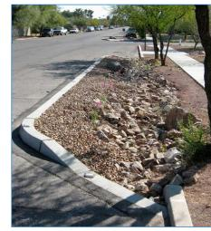
In this just-installed chicane, 4"-8" rock is used in the channel where stormwater will flow rapidly, and 1" gravel covers upslope areas.
