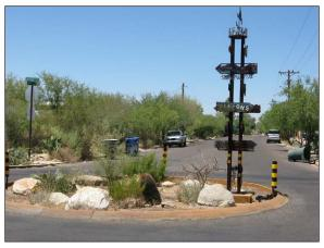
At the top of its sub-watershed, this traffic circle (right) was designed to capture and retain the rain that falls on it.
