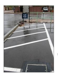
At this University of Arizona parking lot, an unused space happened to coincide with the lot's natural low point. The asphalt was removed and a biorention basin installed. Note concrete header and curb stops. The basin's interior was terraced and shaped to distribute stormwater evenly. Overflow exits the back left corner to the street.
