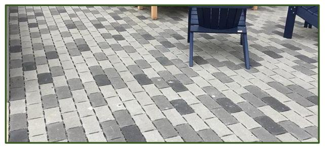
Photograph 5-15. Patio constructed with permeable pavers. (Author & Source: Unknown)
