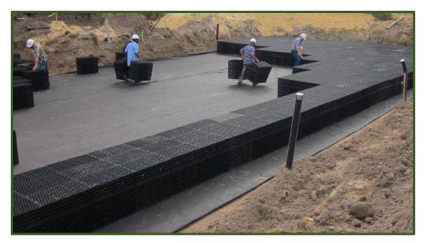
Photograph 5-31. R-Tank® modular system being constructed. (R-Tank, Author & Source: ACF Environmental)
