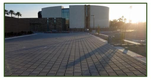
Photograph 5-18. PaveDrain system installation at Franciscan Renewal Center, Paradise Valley, AZ. (Source: Holistic Engineering and Land Management, Inc.)
