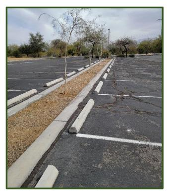
Photograph 1-2. Parking lot draining to median basin with flush curbs at Lake Havasu City Aquatic Center.
