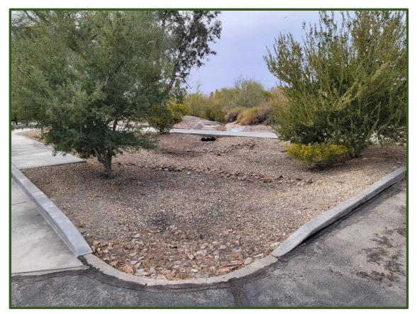
Photograph 1-1. Curb cut with swale and check dams at Lake Havasu City Aquatic Center.
