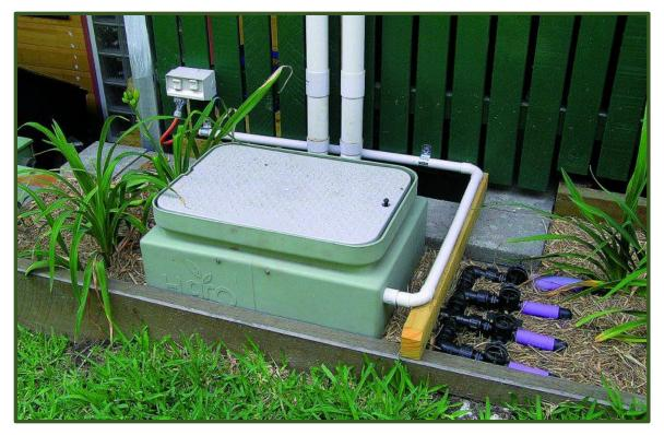
Photograph 5-36. Example greywater irrigation system. (Settling Tank and Components, Author & Source: Renew Organization)
