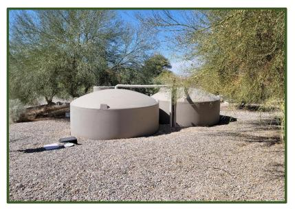
Photograph 1-3. Cisterns capturing rainwater and greywater for irrigation reuse at Street Maintenance Facility.
