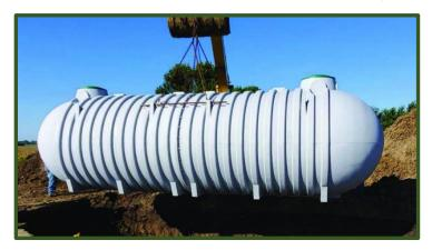
Photograph 5-34. Commercial, underground fiberglass cistern, 10,000 gallons. (Underground Fiberglass, Author & Source: National Storage Tank)
