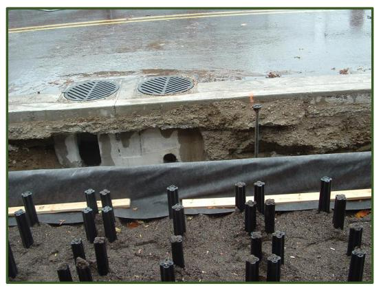
Photograph 5-21. Street catch basins connected to pervious storage media. (Queensway Sustainable Sidewalk Pilot Project, Author: City of Toronto, Source: Sustainable Technologies)
