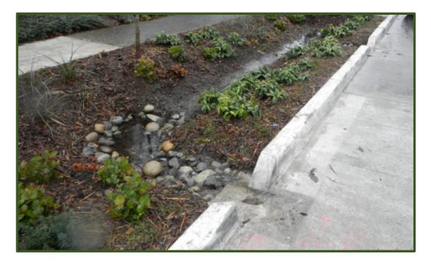
Photograph 5-39. Sediment trap at roadway curb cut. (Author & Source: NACTO)
