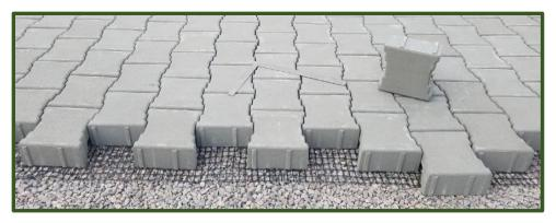
Photograph 5-16. PaveDrain system at Franciscan Renewal Center, Paradise Valley, AZ – spacers, mesh, rock bedding. (Source: Holistic Engineering and Land Management, Inc.)
