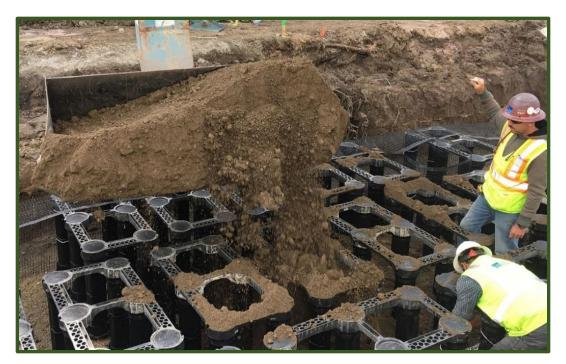
Photograph 5-20. Silva Cell system installation. (Silva Cell Trenching, Author & Source: Deeproot)
