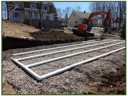
Photograph 5-30. Perforated pipe distribution system example. (Author & Source: Wikipedia/Nonztp)
