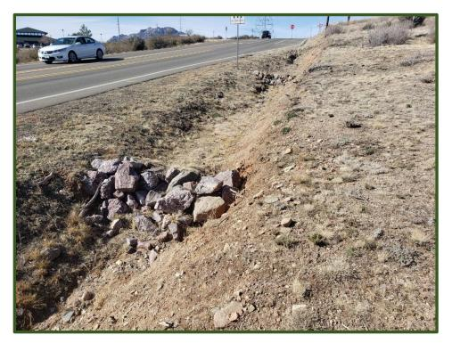
Photograph 5-4. Check dam example, Yavapai County roadway swale. (Source: HELM)
