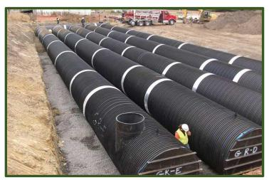
Photograph 5-35. Underground steel-reinforced polyethylene cistern backfilled with 50 percent stone. (Author: Greg Kowalsky and Kathryn Thomason, Source: Contech Engineered Solutions)
