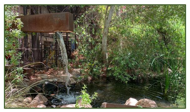
Photograph 5-38. AC condensate refilling pond and infiltrating into aquifer (CAPLA Underwood Garden, Author: Bill Timmerman, Source: Green Infrastructure Digest)
