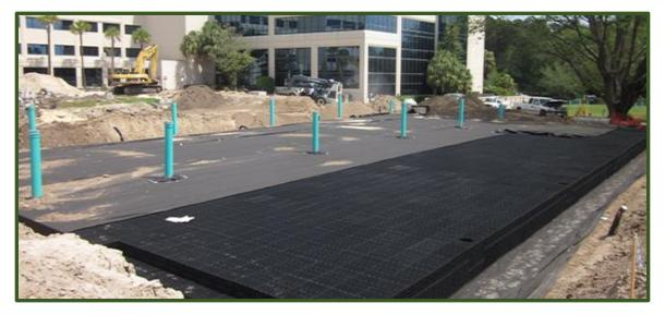
Photograph 5-32. R-Tank® modular system before backfilling. (R-Tank, Author & Source: ACF Environmental)
