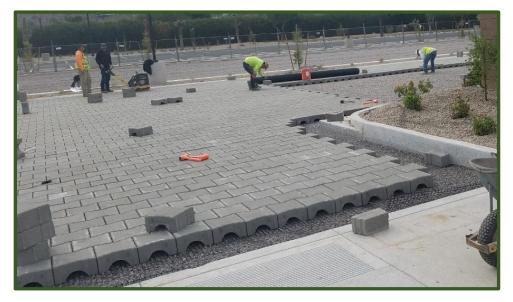
Photograph 5-17. PaveDrain system at Franciscan Renewal Center, Paradise Valley, AZ – installation and arch design. (Source: Holistic Engineering and Land Management, Inc.)
