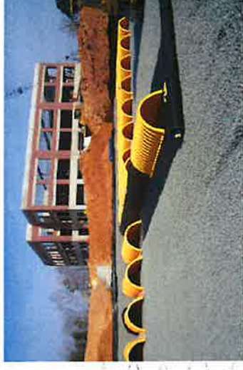
Example of an underground Retention facility.
